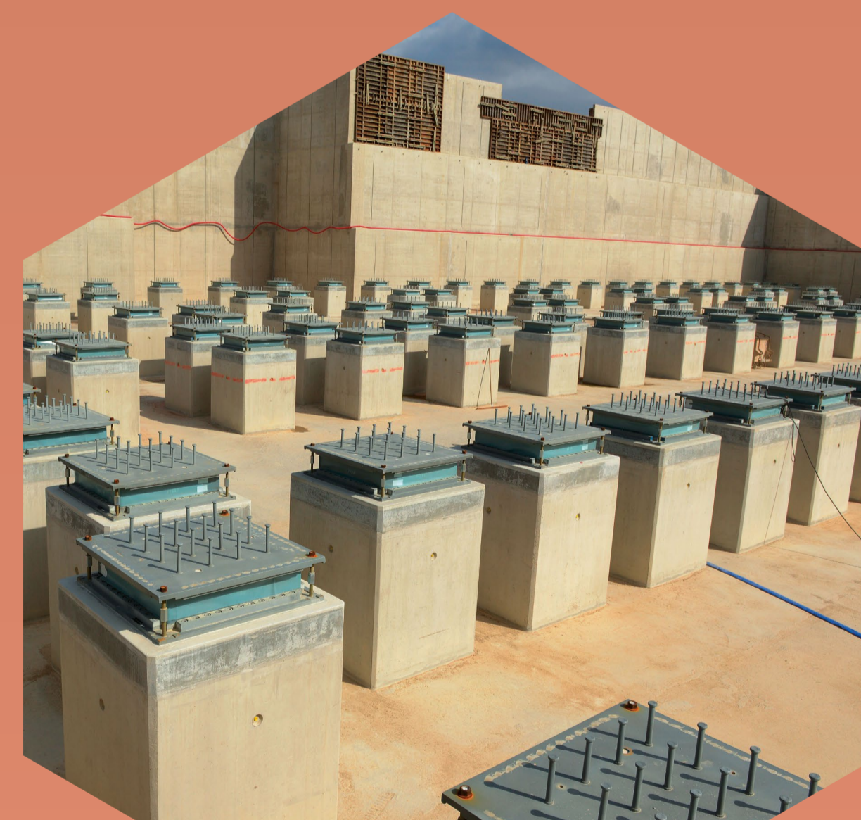
Concrete blocks fitted with earthquake-resistant pads. The pads are made of rubber and metal. They can limit the accelerations and shear forces associated with ground movements during an earthquake.
