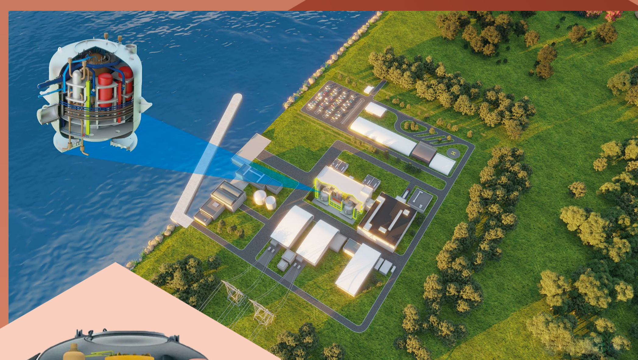
NUWARD™ reactor vessel and containment in the overall view of the main nuclear building.
