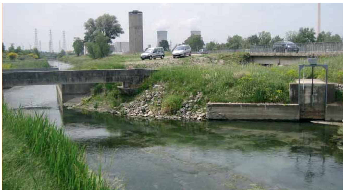
Figure V.25 - Right-bank counter-ditch upstream of the Tricastin nuclear site
