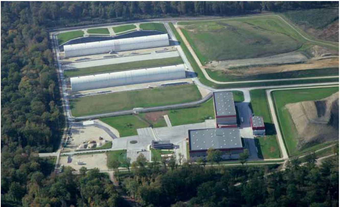
Figure V.140 - CSTFA waste disposal facility at Morvilliers
