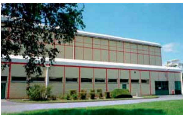
Figure V.134 - Somanu plant workshop ("hot workshop")
