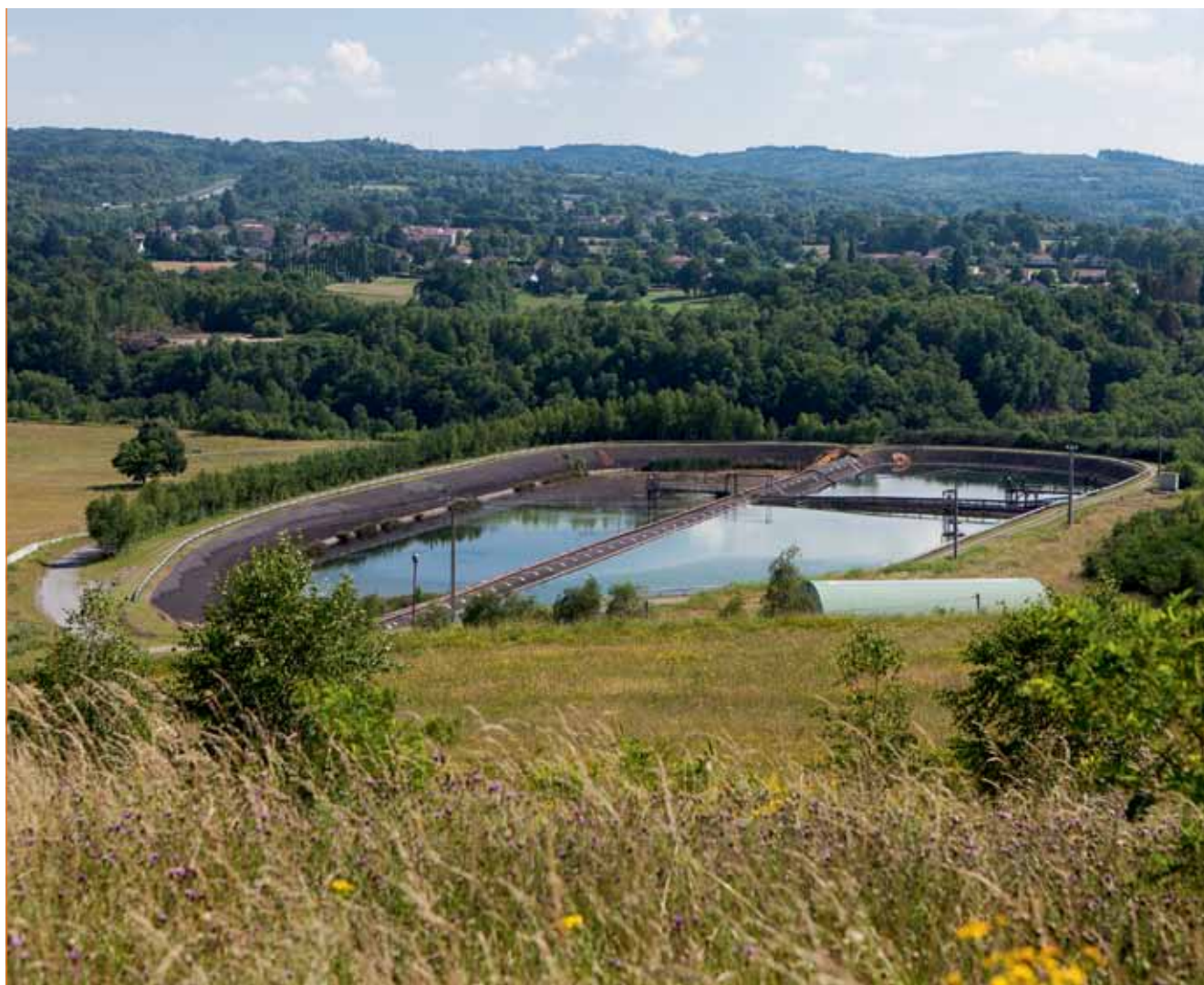
Figure V.4 - Pond for drain water from the uranium mine tailings disposal facility at the Bessines-sur-Gartempe site
