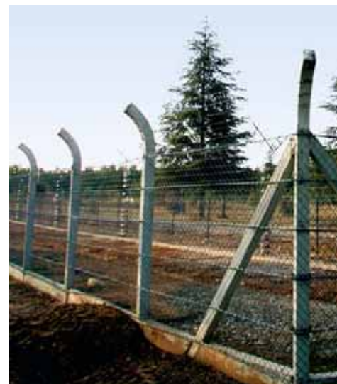
Physical protection barrier.
