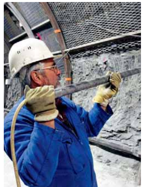
Inserting instrumentation into a borehole.
