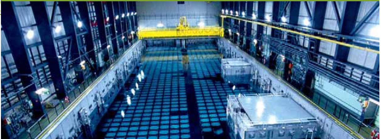
Fuel pit at the La Hague plant.
