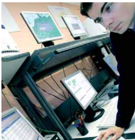
Warning network remote monitoring room in Le Vésinet (Yvelines).
