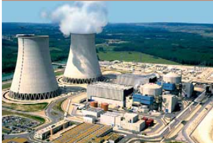
The Institute's Crisis Centre was activated on 30 September 2005 following a water leak at the Nogent-sur-Seine power plant.
