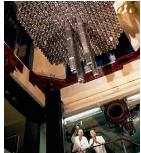
Bottom view of the MASURCA reactor, during insertion of fuel rods.
