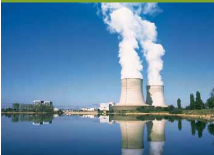
The site at Saint-Laurent-des-Eaux. The first CLI was mobilised to set up the pilot project conducted in the Loire basin.
