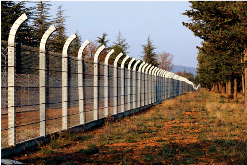
Figure 14. Physical protection barrier, Cadarache, France. © Olivier Seignette/Mikaël Lafontan/IRSN.
