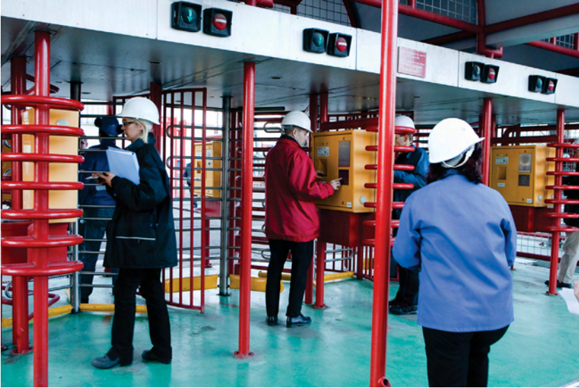
Figure 15. Access control system at the Fessenheim site, France. © Noak/Le Bar Floréal/IRSN.
