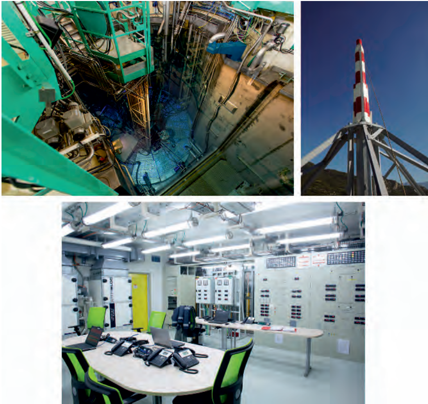
Figure 10.9. Three measures selected for the RHF at Grenoble after the Fukushima Daiichi accident, all designed and sized for extreme earthquakes and flooding: on the top left, the pool inlet elbow of the groundwater supply system. © IRSN; on the top right, the seismic depressurization system stack positioned on the dome of the metal containment. © ILL; at the bottom, the PCS 3 emergency control room. © Jean-Marie Huron/Signatures/IRSN.
