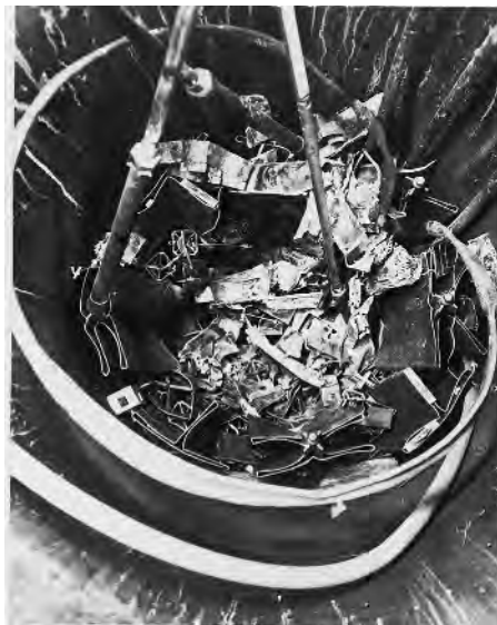
Figure 8.1. View of the SL-1 reactor core after the reactivity accident in 1961, three of the rod mechanisms are visible. @ INL.
