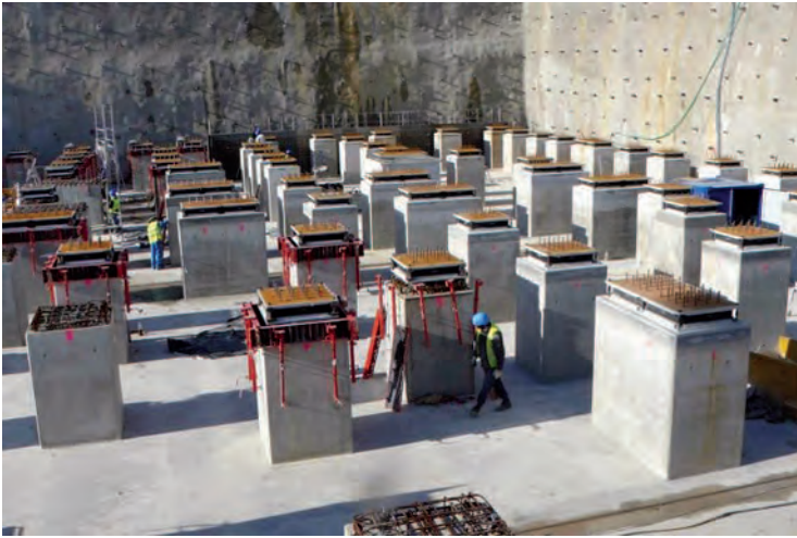
Figure 7.11. View of aseismic bearing pads during construction of the Jules Horowitz reactor (2009), from “ Le Blog des Énergies ”. © DR.
