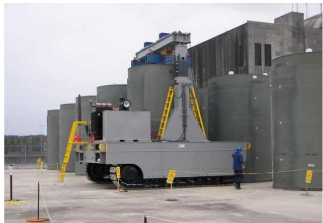
Figure 32: Photo of a storage facility using the HI-STORM 100 concept
