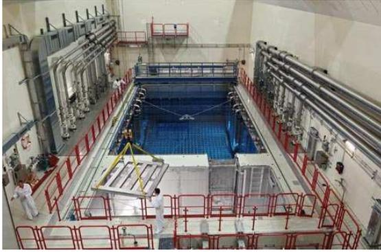
Figure 10: Photo of the pool of the 'fuel storage building' at the Gösgen NPP (Switzerland)
