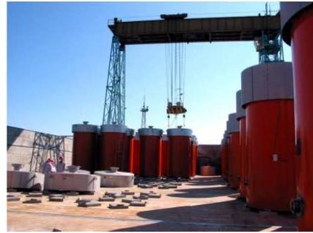
Figure 54: Storage in CASTOR® casks on the Ignalina nuclear power plant site (Lithuania)
