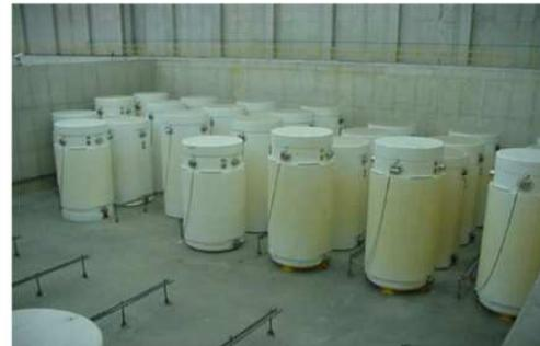
Figure 40: Photo of TN®24 DH casks stored in the dry storage building on the Doel site (Belgium)
