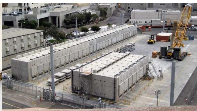
Figure 22: Photo of a NUHOMS<sup>®</sup> module storage facility on the San Onofre site (USA)
