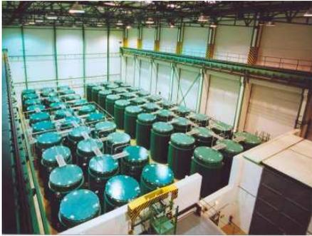
Figure 53: Storage in CASTOR® casks on the Dukovany nuclear power plant site (Czech Republic)
