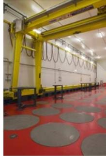
Figure 61: Photo of the top of the storage pits at the HABOG facility (Borsele - Netherlands)
