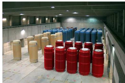
Figure 66: Photo of the interior of the centralised storage facility on the Gorleben site (Germany)
