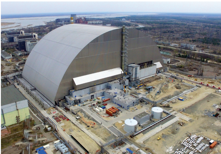
Figure 34.3. The new sarcophagus after installation – photograph taken in 2017. EBRD.
