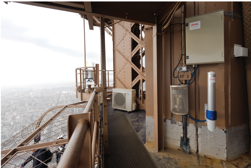
Figure 38.2. Téléray probe installed on the Eiffel Tower in Paris. Arnaud Bouissou/MEDDE/IRSN Media Library.
