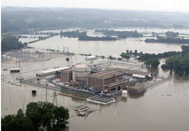
Figure 37.5. In June 2011, high river levels in Missouri caused flooding at the Fort Calhoun nuclear power plant in the USA. Nati Harnik/AP/SIPA.
